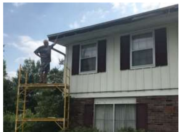
Tom Henning on the Scaffolding
